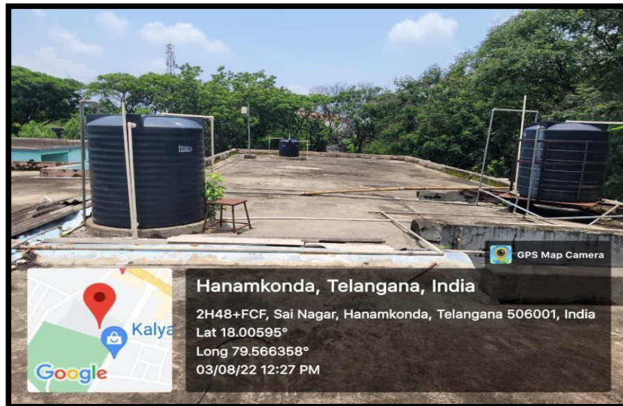
Water Tanks available in the College Campus
