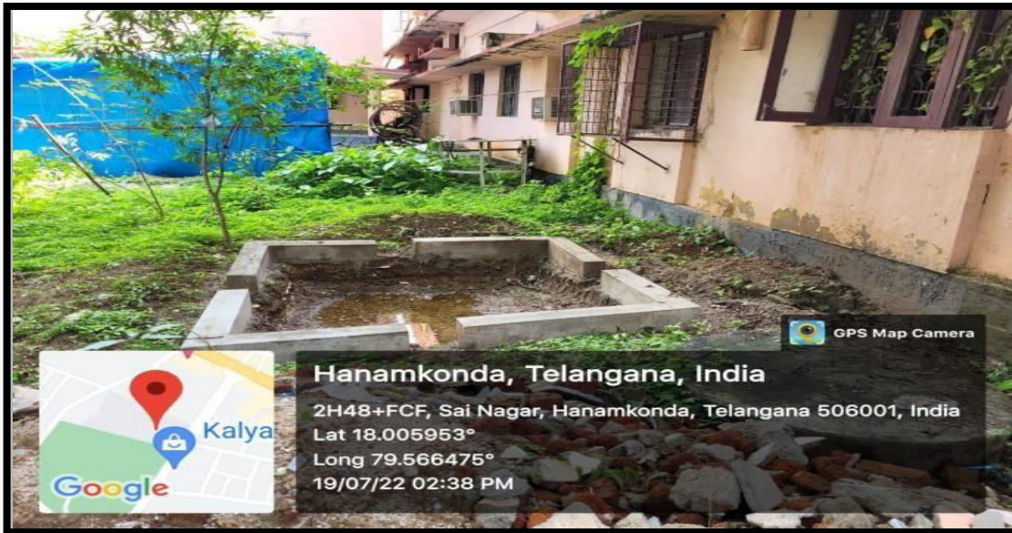
Water Harvesting pits near Main building
